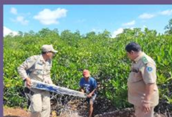
The installation of demarcation poles in the mangrove conservation areas
